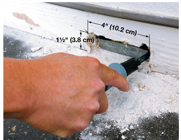
Cut cable access hole in wall
